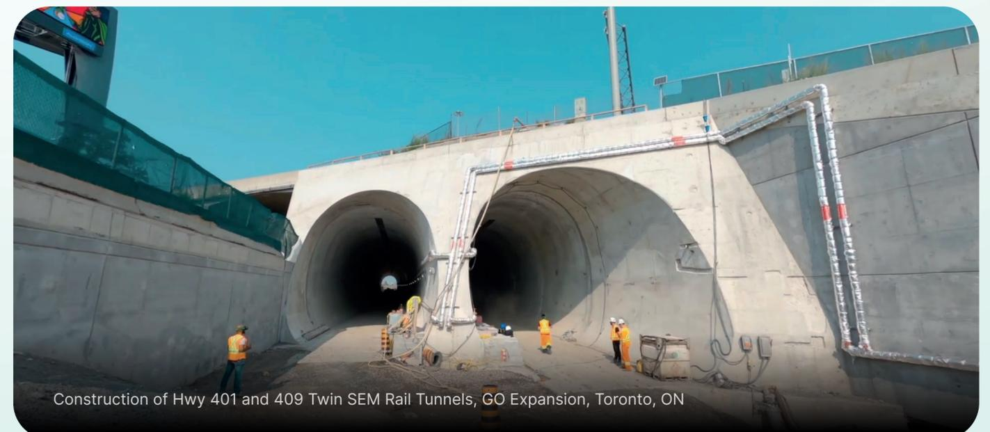
Construction of Hwy 401 and 409 Twin SEM Rail Tunnels, GO Expansion, Toronto, ON
